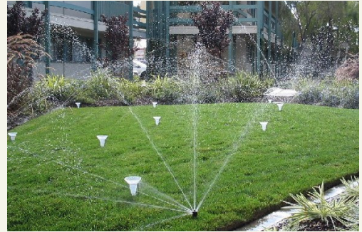
When auditing an irrigation system, set out containers in one station as directed in Step 5.
